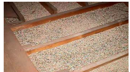
Vermiculite insulation between attic joists
