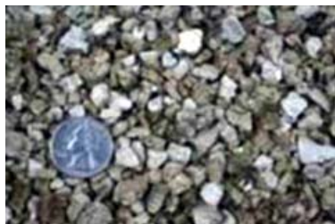
Typical vermiculite insulation
