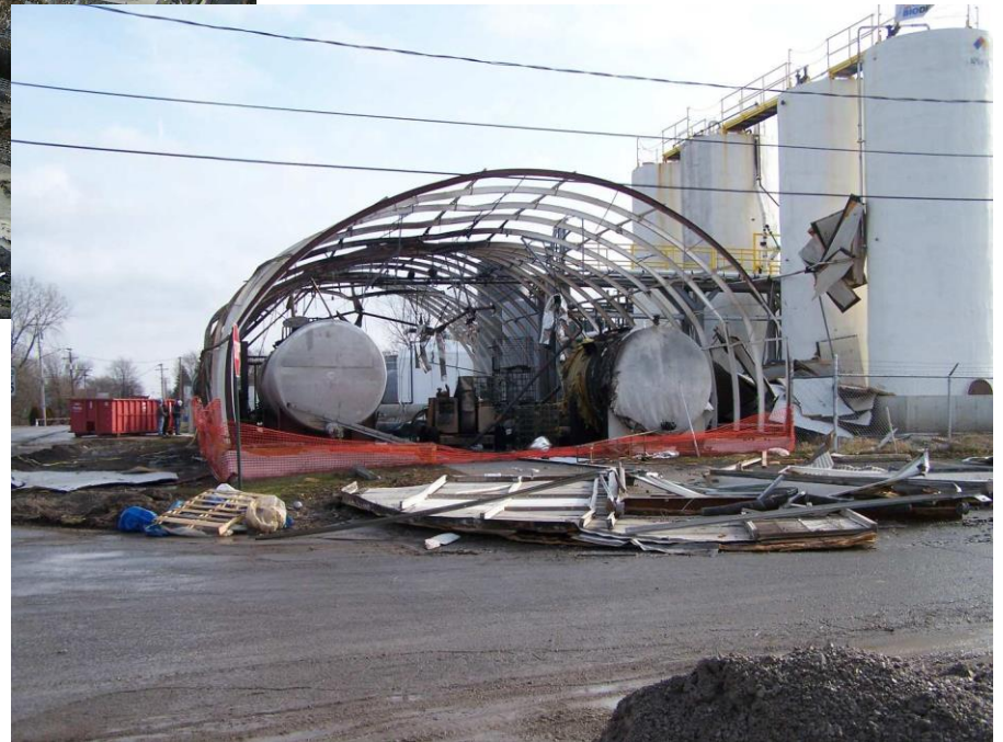
Release came out of structure with FF water
