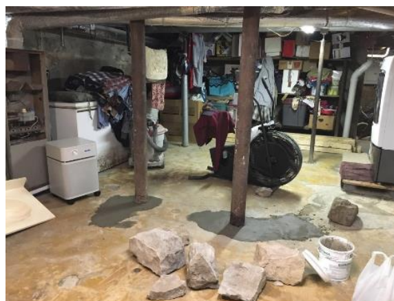
Figure 9-3. Holes in Floor Sealed with Hydraulic Cement
