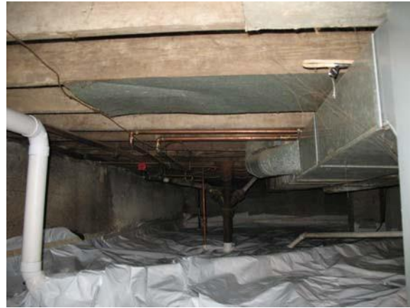
Figure 9-22. Piping in Crawl Space
