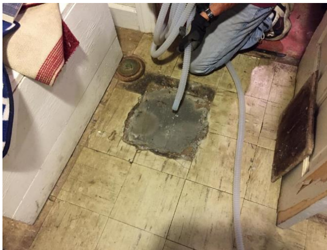
Figure 9-5. Dry Sump After Filling with Concrete
