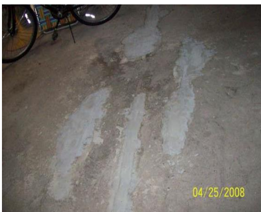
Figure 9-2. Cracks in Floor Sealed with Hydraulic Cement
