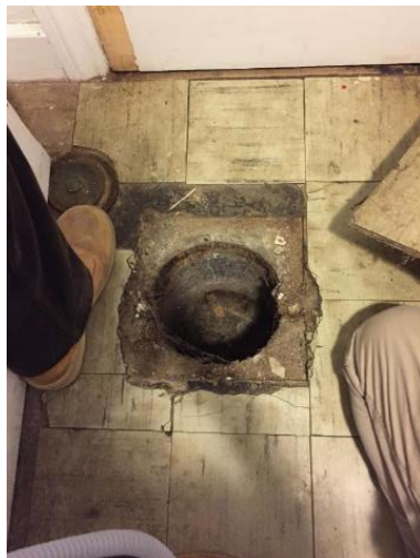
Figure 9-4. Dry Sump Prior to Filling with Concrete
