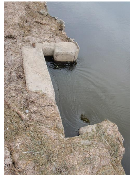
Culvert opening on north side of Dam 8
