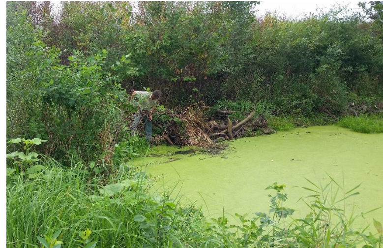
Culvert inlet, blocked by vegetation
