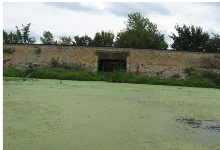
Box culvert under railroad bridge on east shore of marsh
