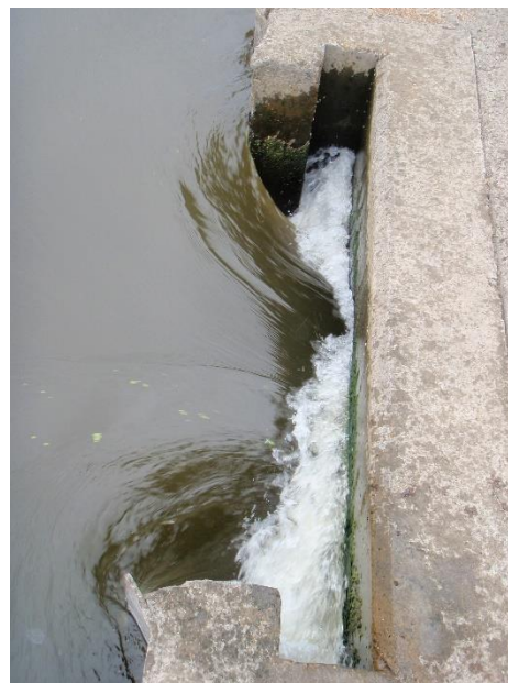
Culvert opening on north side of Dam 8
