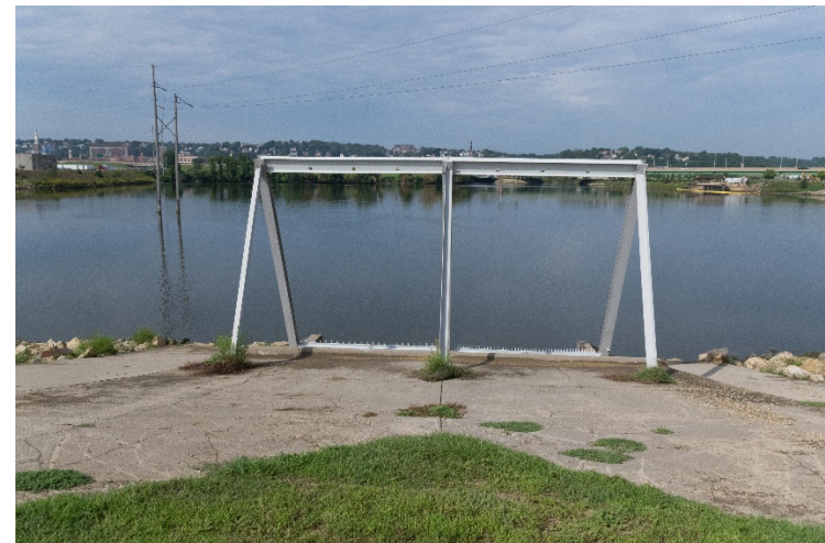
Top of culvert gate
