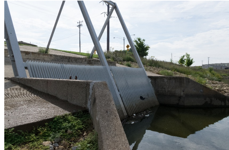
Culvert inlet
