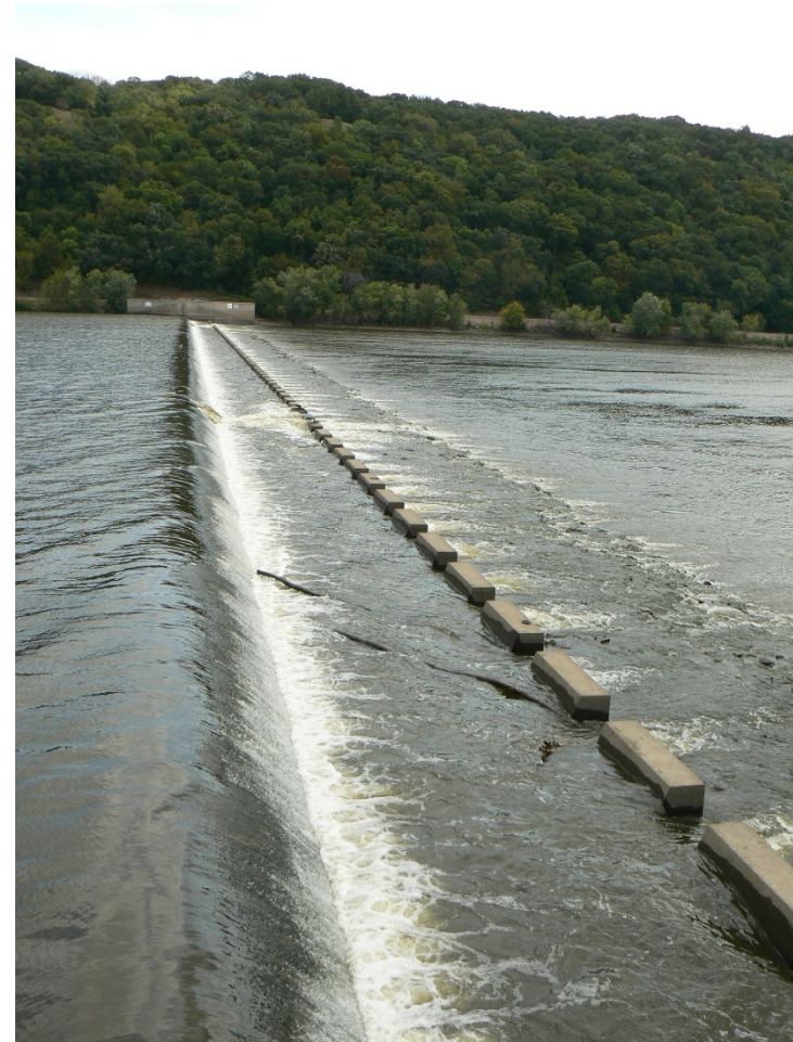
Spillway overtopped in higher water
