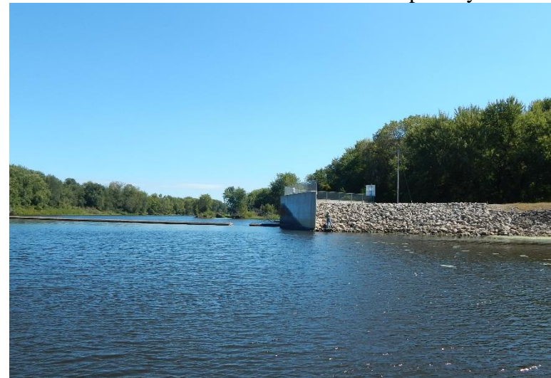
West end of spillway, note notch near wall
