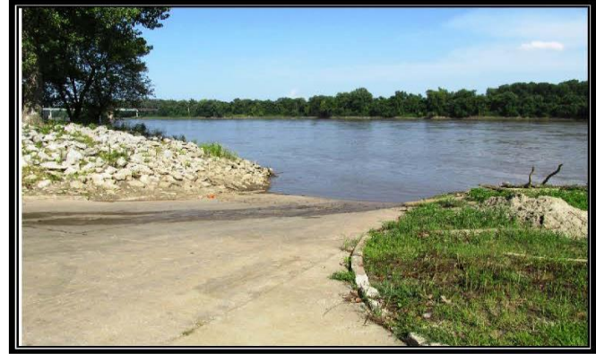
Looking East – Down concrete boat launch
