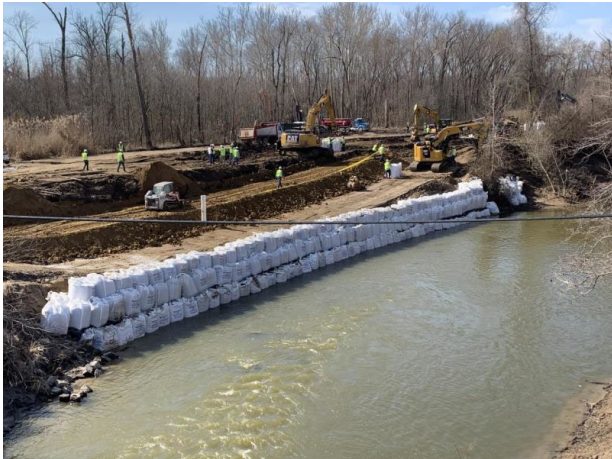
March 17 Shoreline protection of pipeline release point
