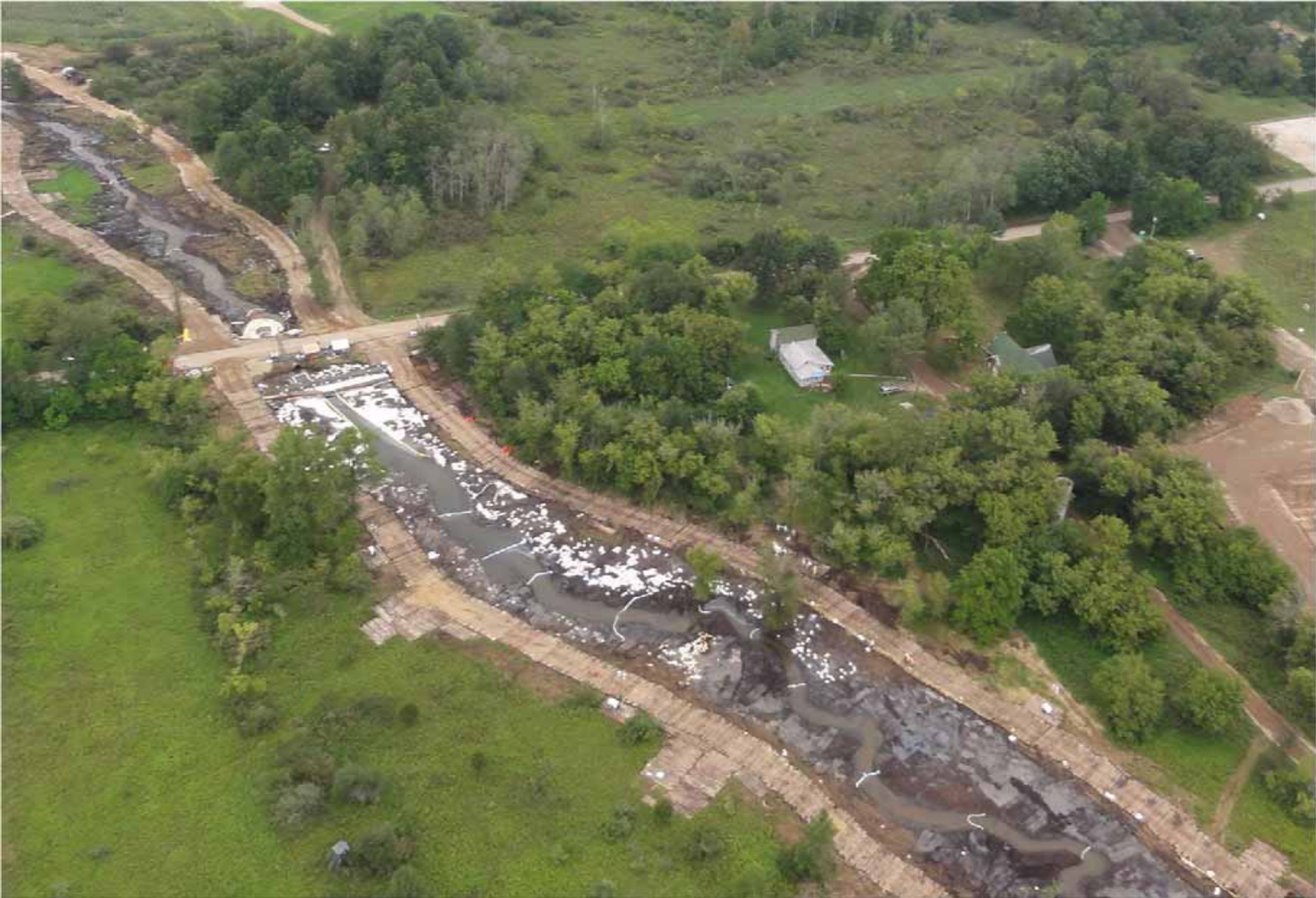
To access the creek in order to remove contaminated soil, swamp mat roads were established. Note white oil pads placed to absorb oil.
