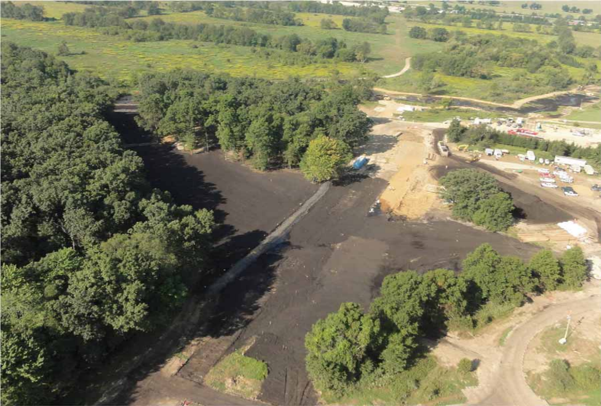
After four weeks, contaminated land located by the pipeline break was backfilled with clean soil.
