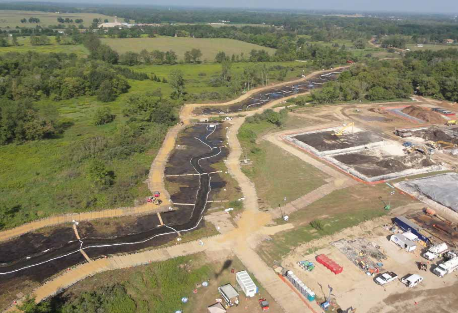
Talmadge Creek after soil scrapping was completed. Contaminated soil staging pads visible on the right side of the picture.
