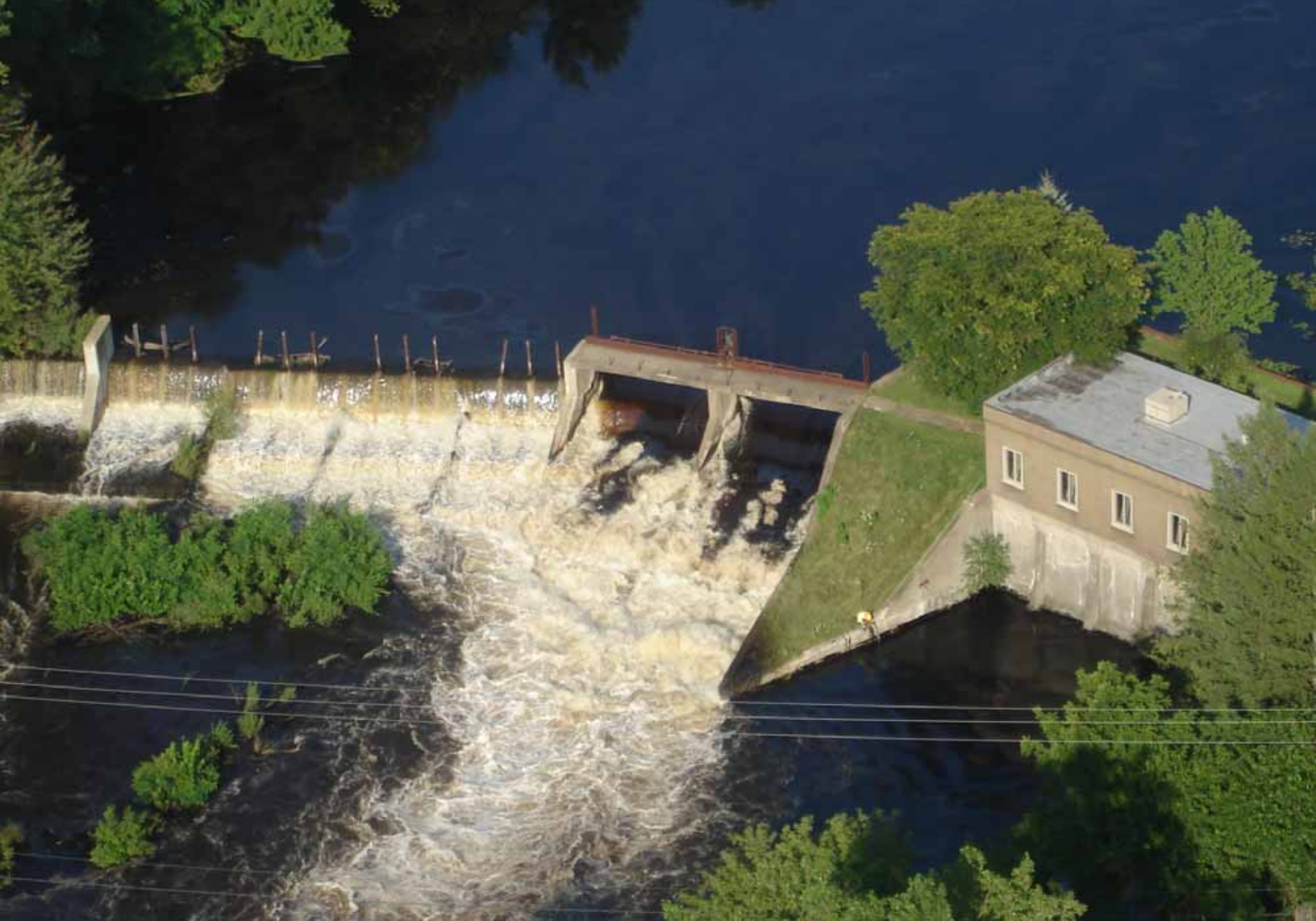
July 26, 2010, Ceresco Dam: note the oil flowing over the dam.
