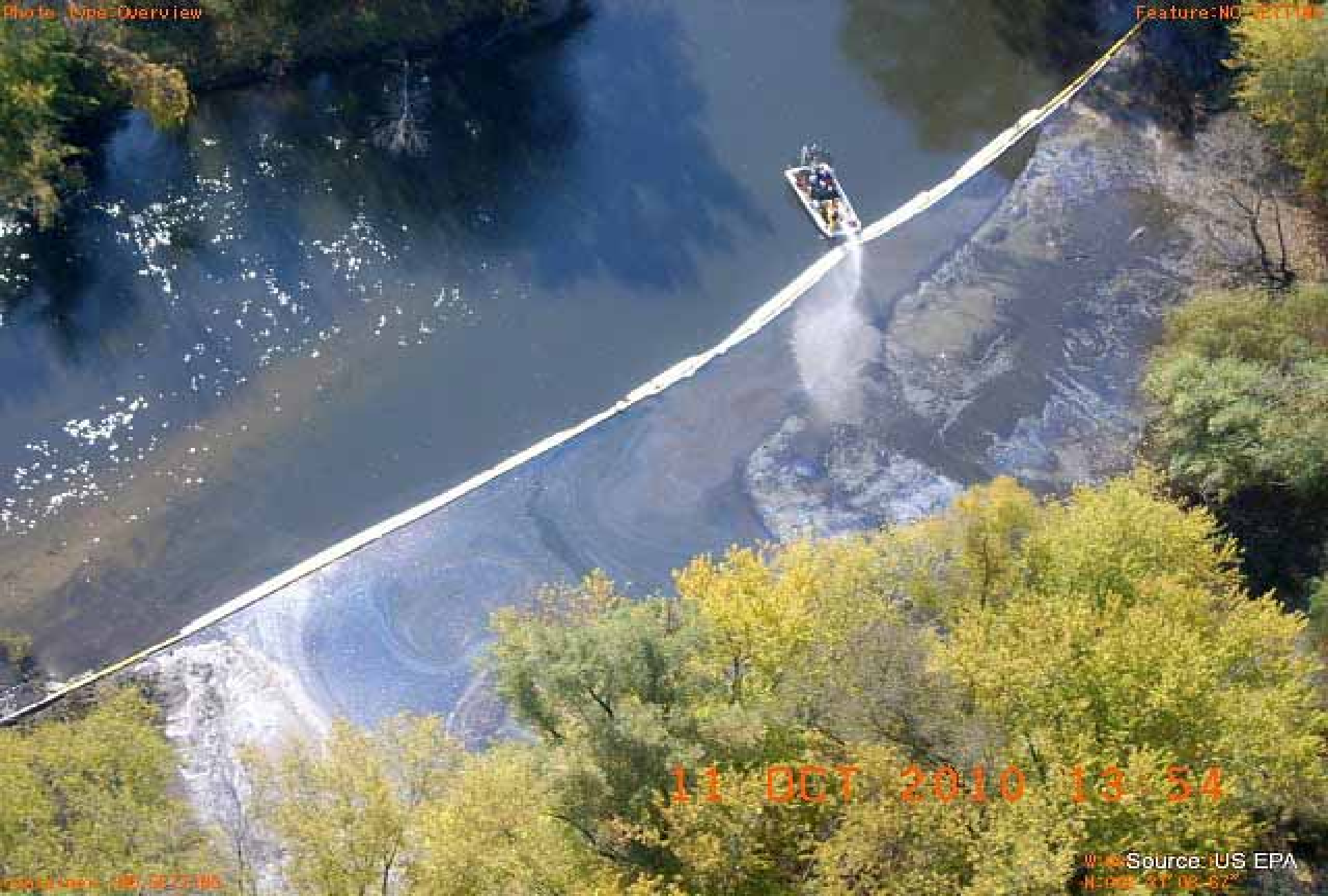
Example of submerged oil aeration, flushing, and recovery. Sediment is agitated to reintroduce oil to the surface so it can be collected.
