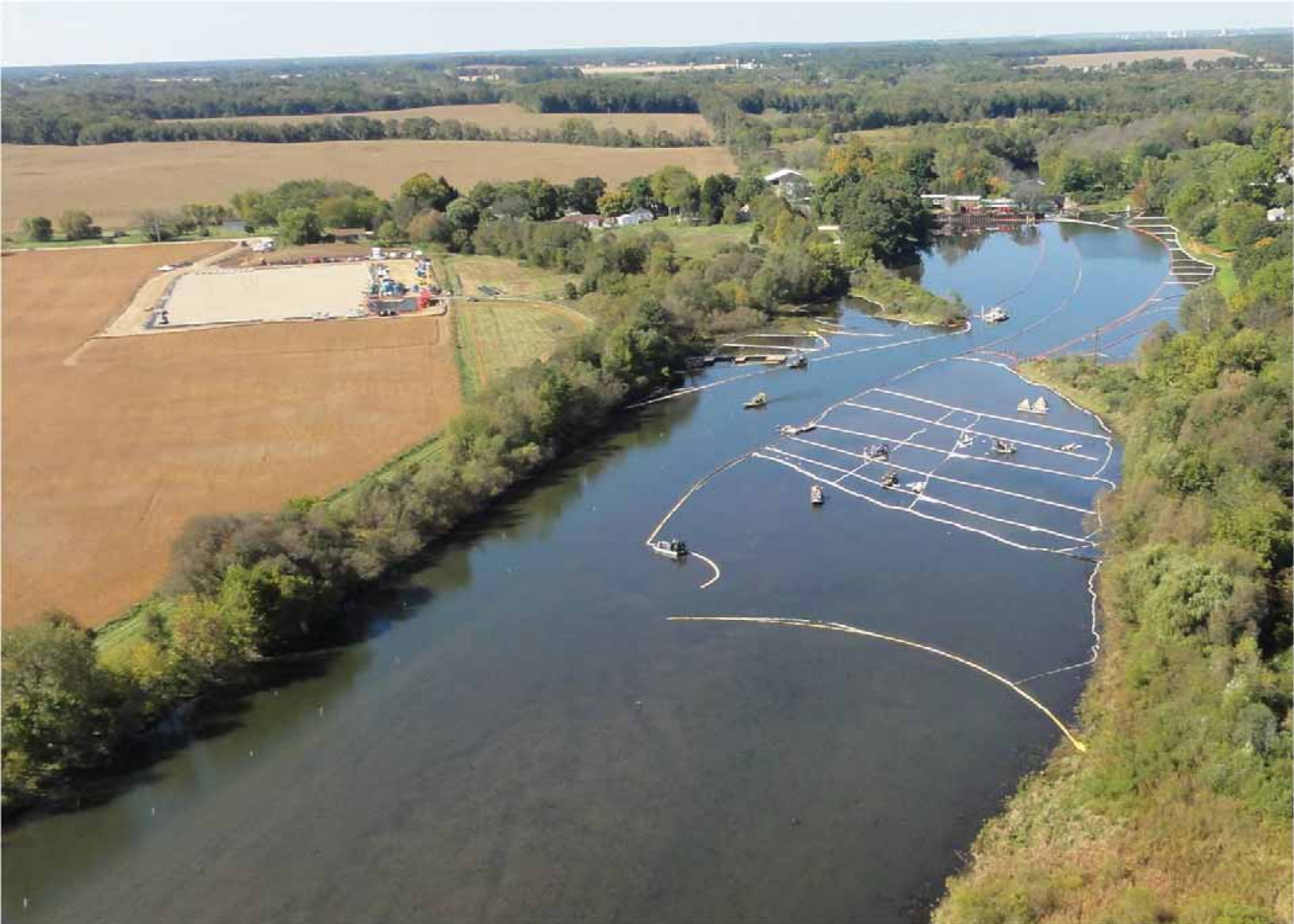
October 2010: submerged oil cleanup started upstream of Ceresco Dam.
