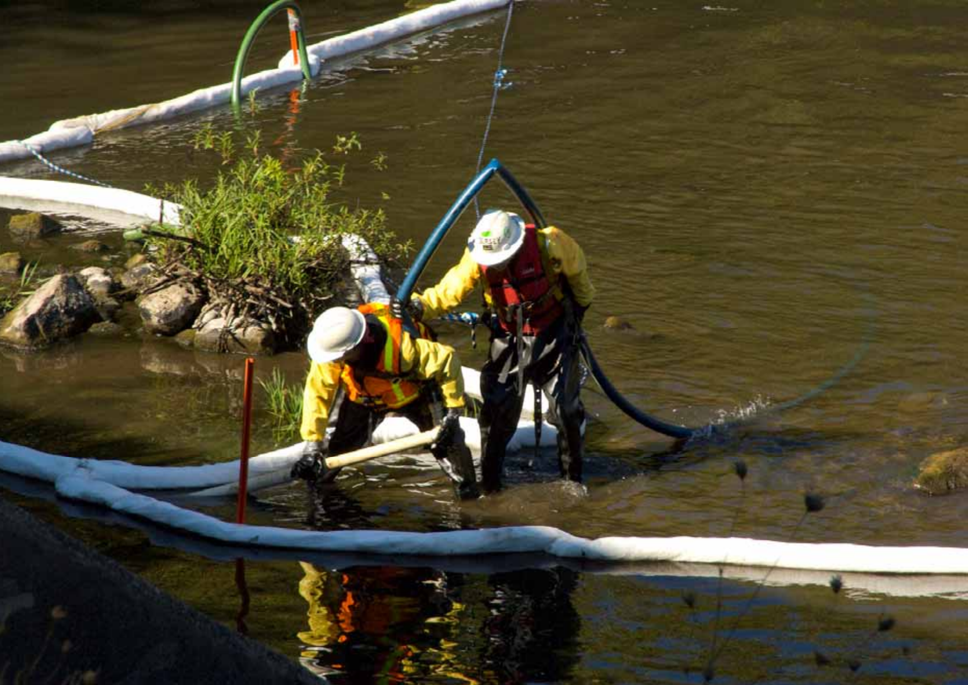
Close-up shot of aeration activities.
