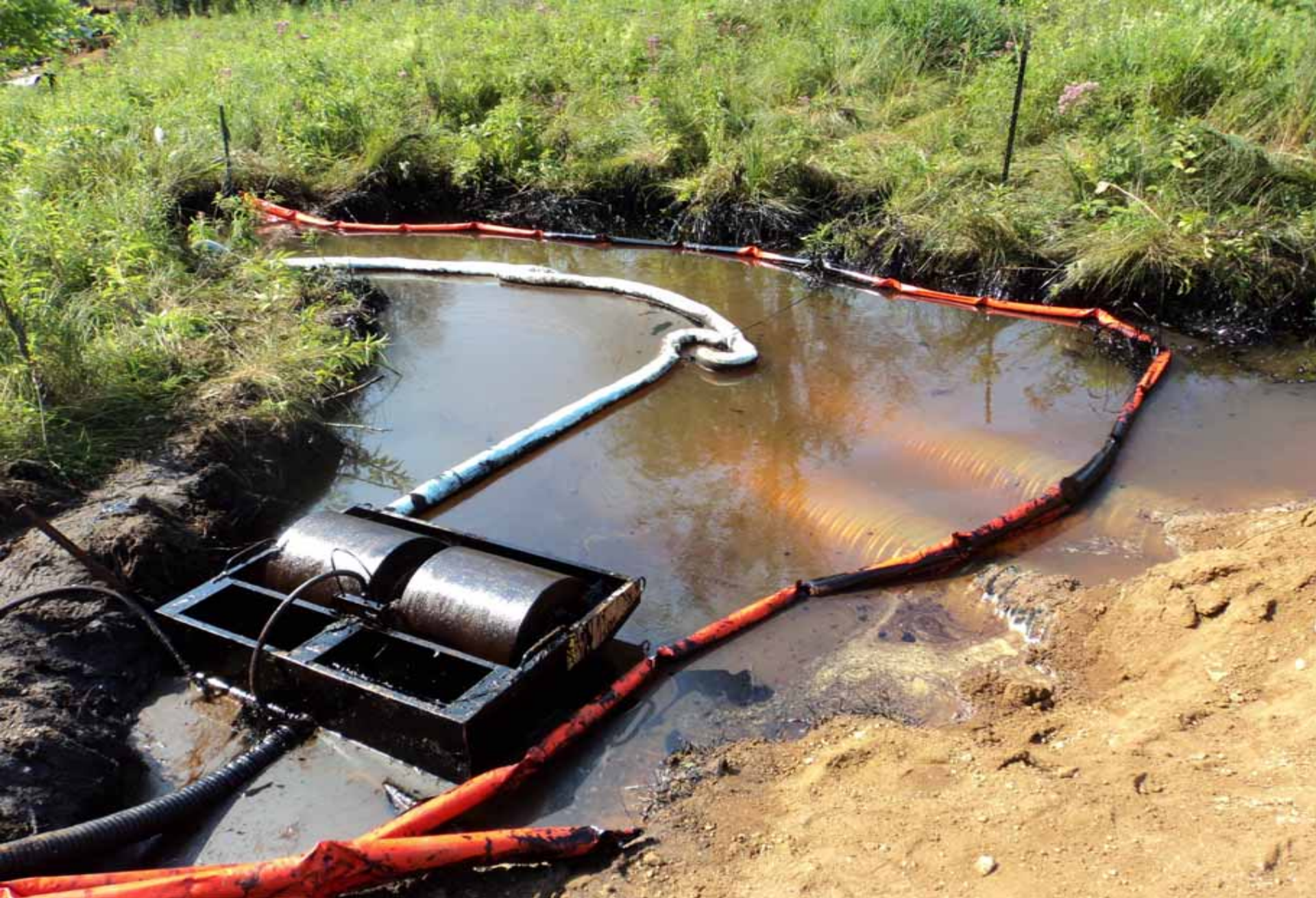
Initial containment measure in the creek includes skimmers, containment booms, and siphon dams.
