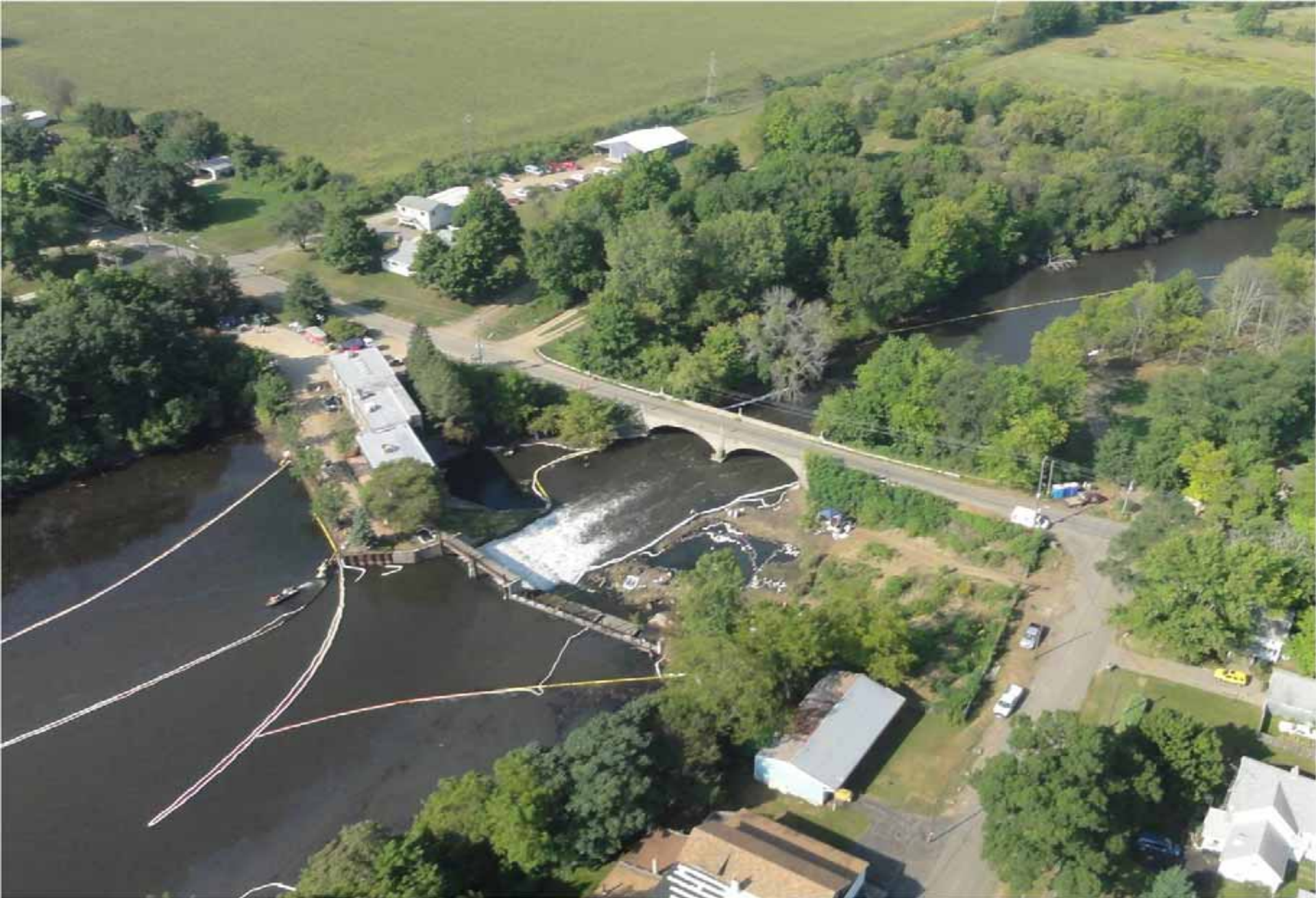
Containment booming established to control vegetation sheening upstream of Ceresco Dam.
