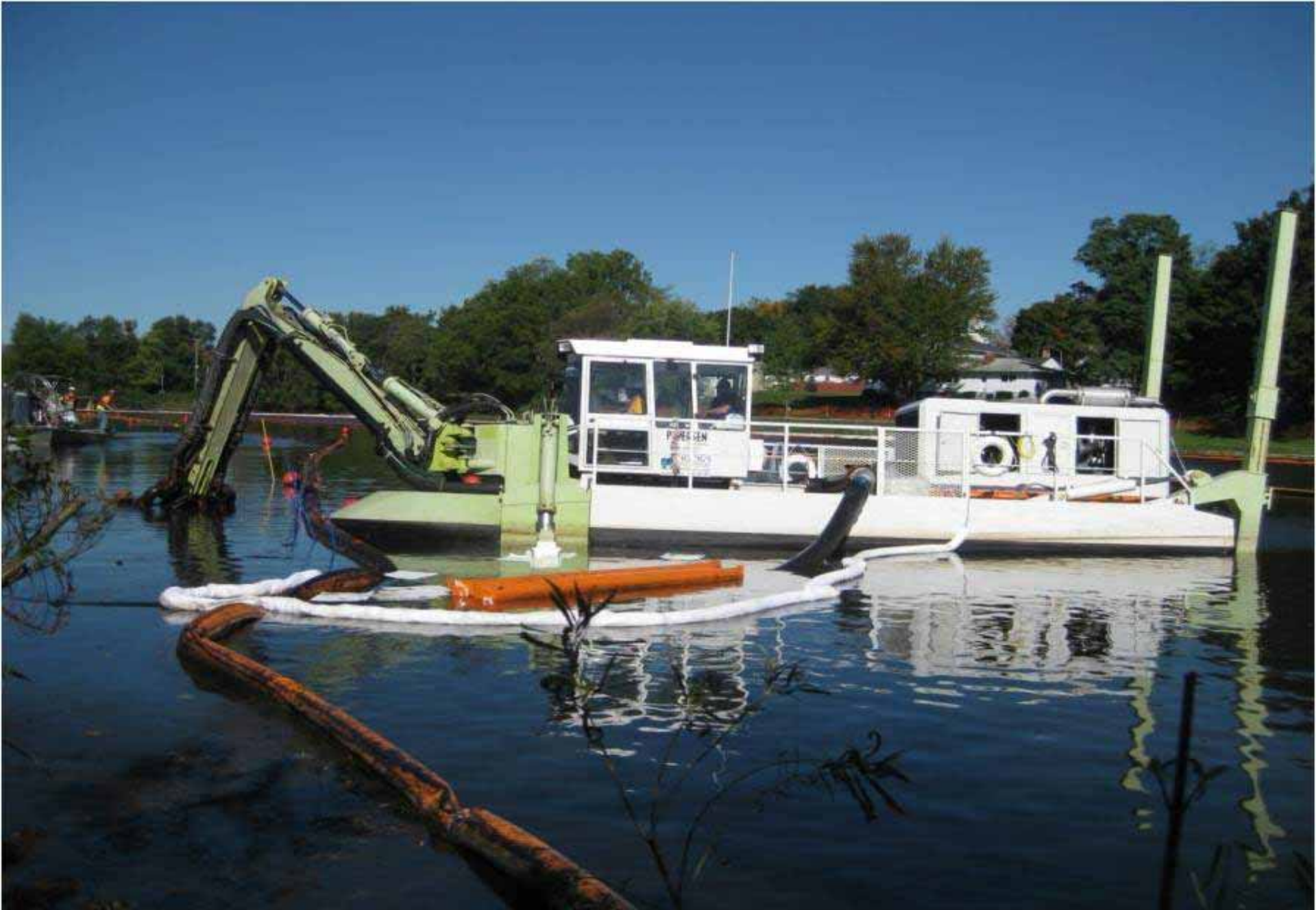
Amphibex dredge used to remove approximately 18 inches of sediment from upstream of Ceresco Dam.
