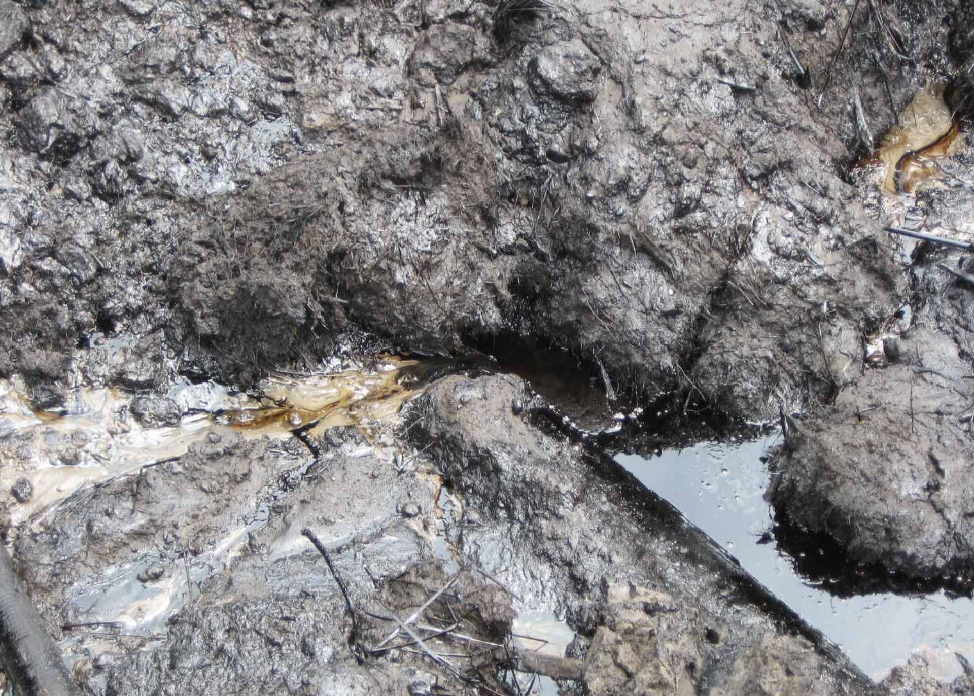
Exposed pipeline during the first week of the oil spill response.
