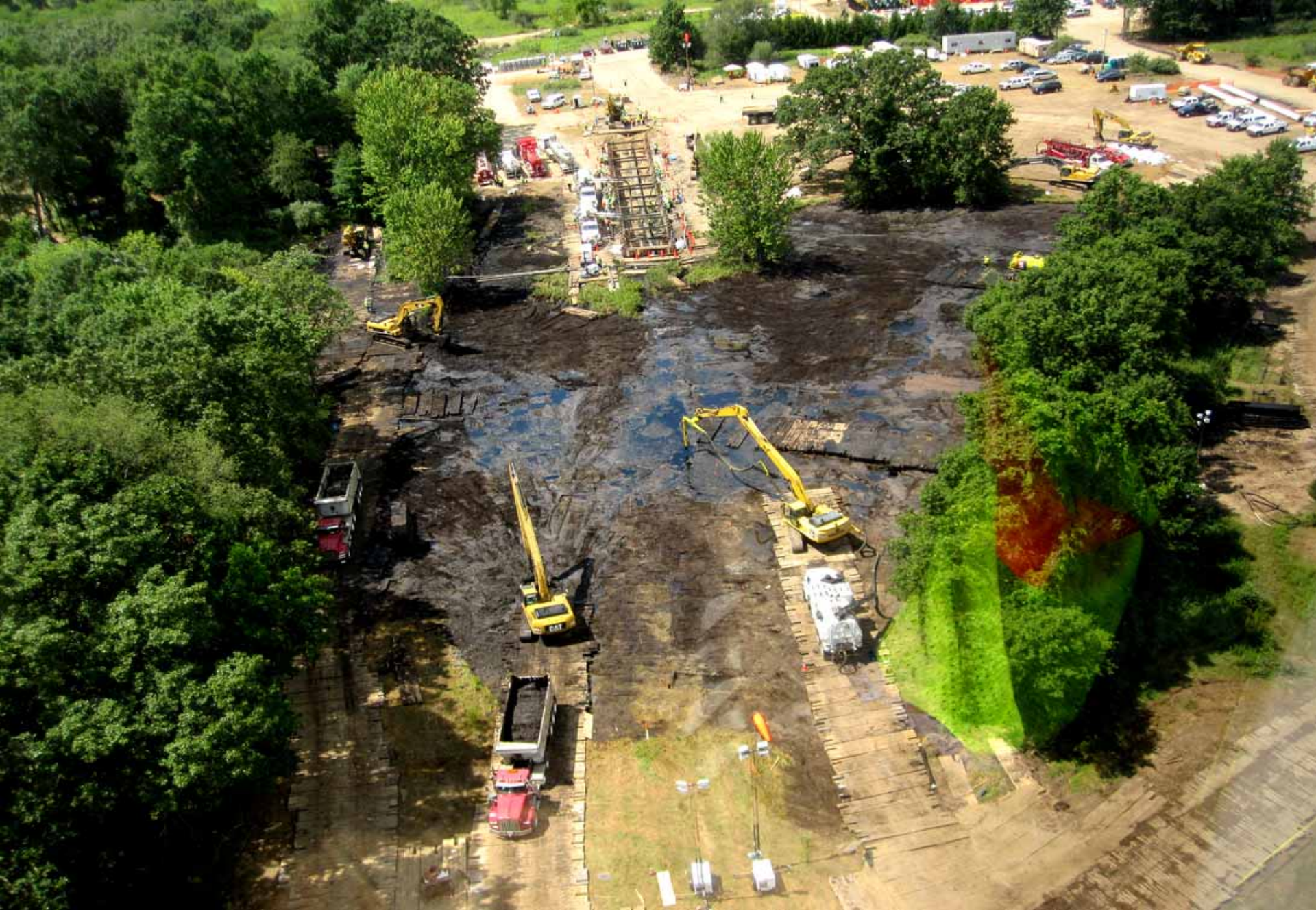
Second week of contaminated soil cleanup near the pipeline break.
