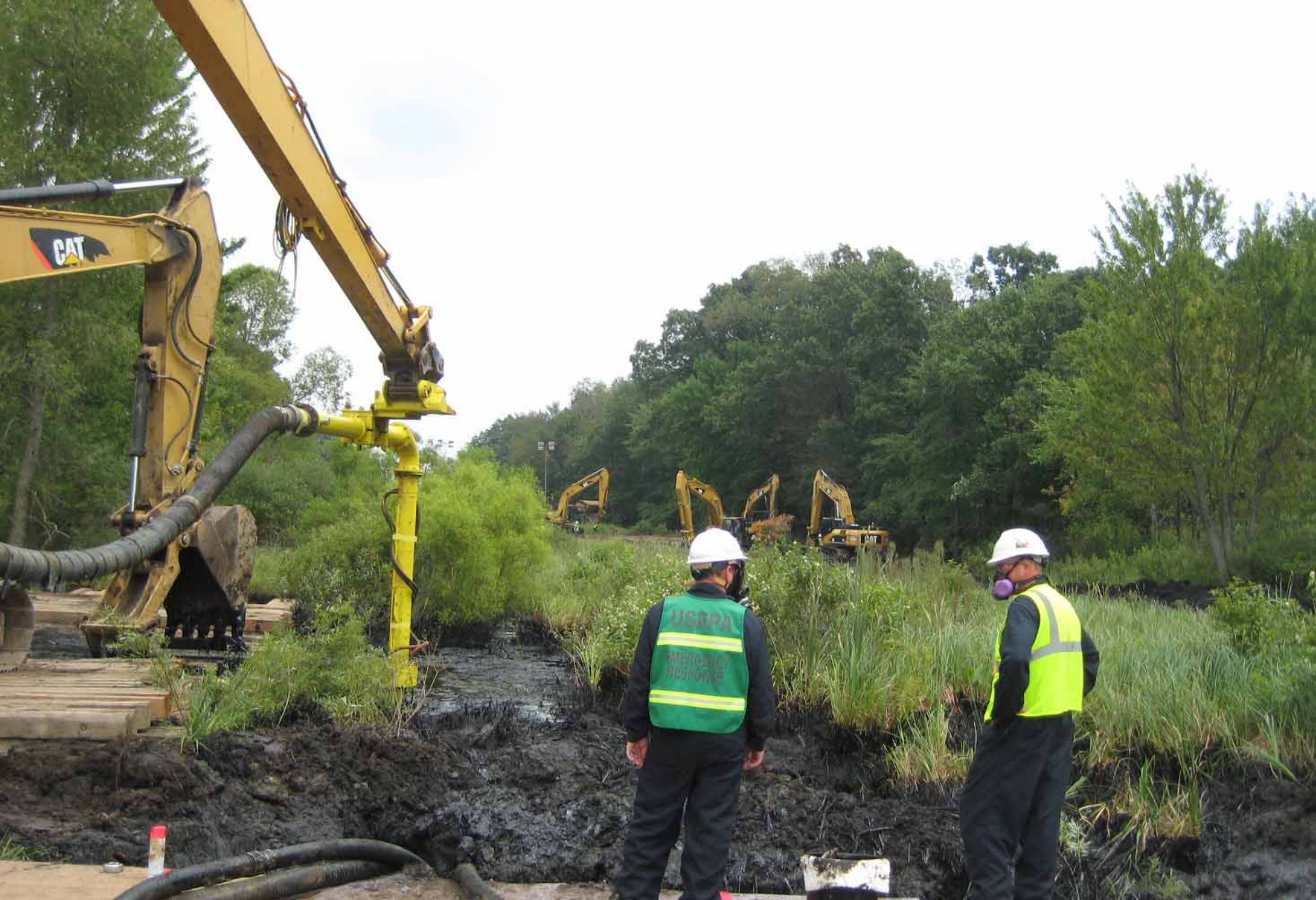
Initial cleanup of a 5-acre contaminated zone in the pipeline break area. Photo shows a dewatering operation.
