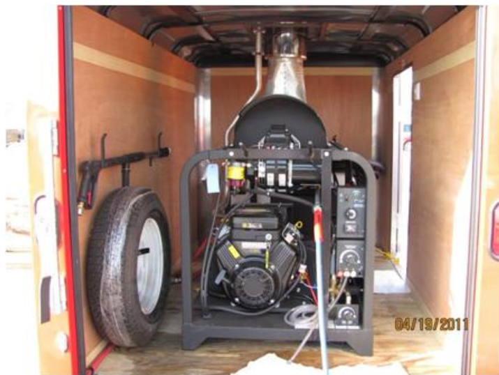
Steam Generator in Trailer
