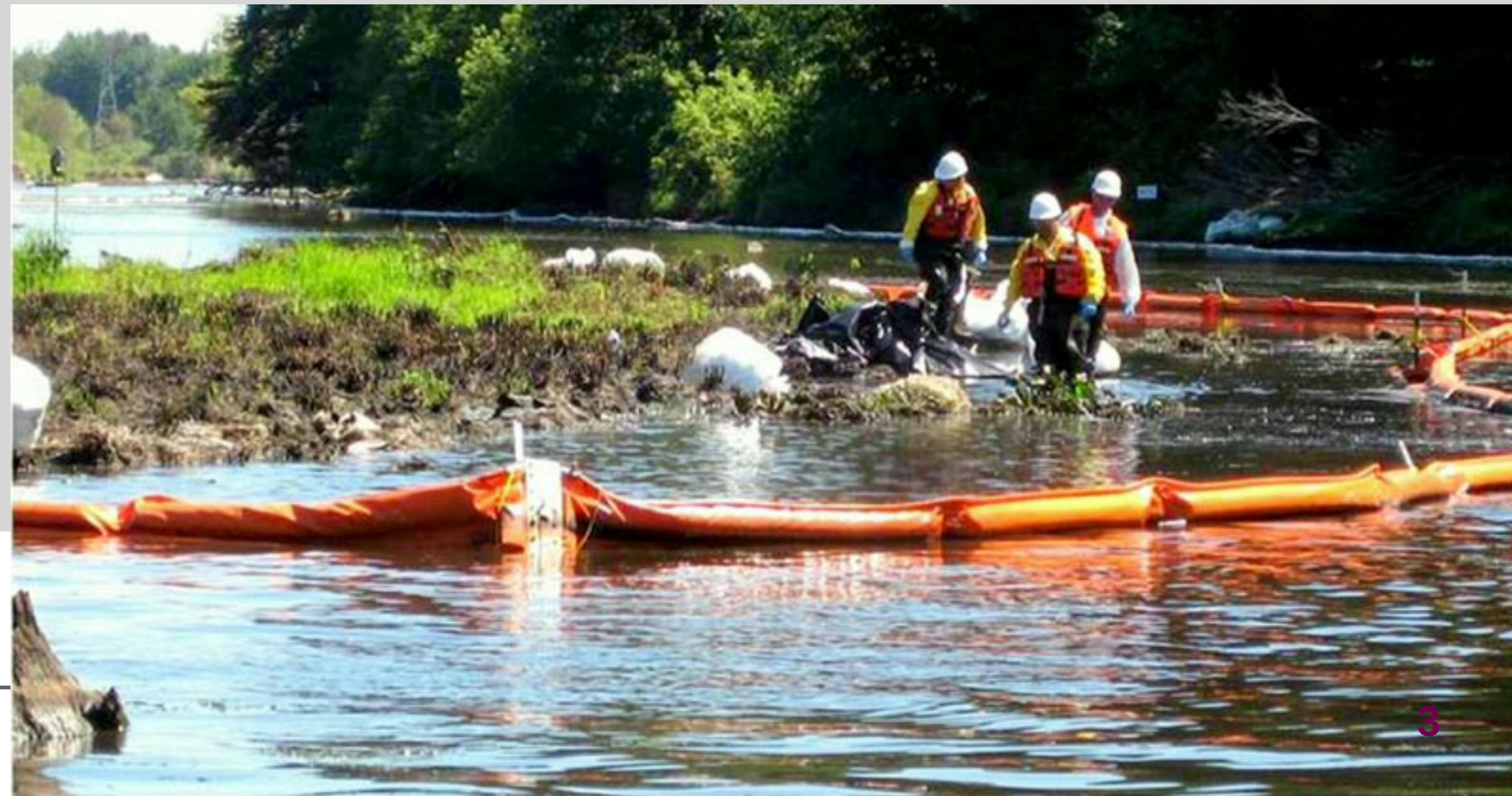
Containment of an oil spill with a boom on the Kalamazoo River, 2010. Photo from www.oilandwaterdontmix.com .
