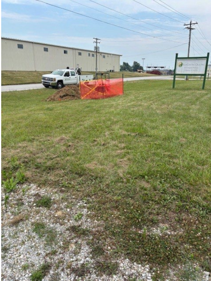
Waterloo sanitary sewer cut off location.
